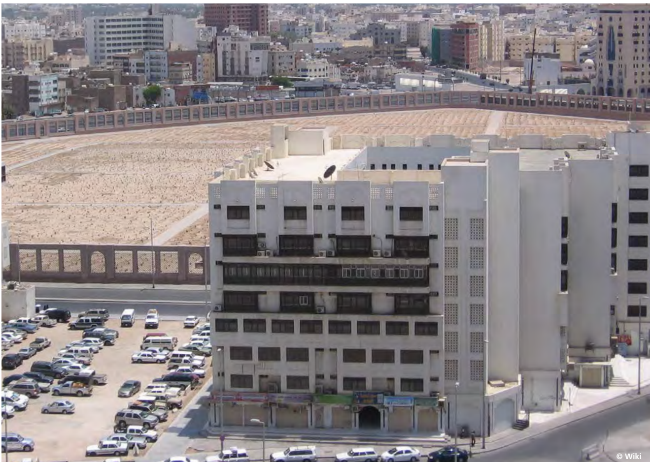
The Al-Baqi Cemetery is an important space within Madinah urban structure
