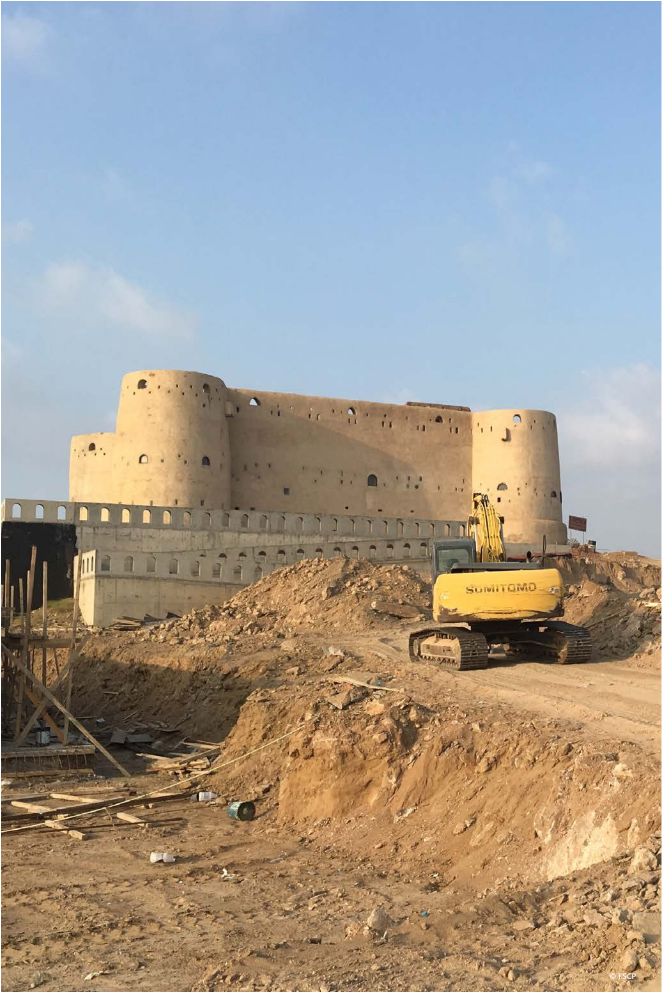
The Jazan Ottoman castle under renovation
