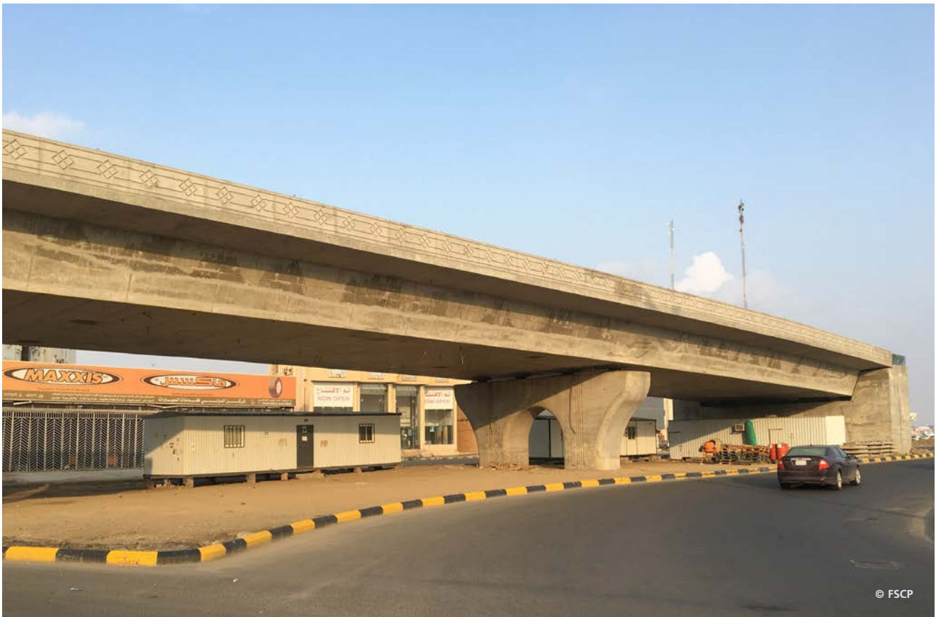
Bad designed infrastructure creates divisions in the city
