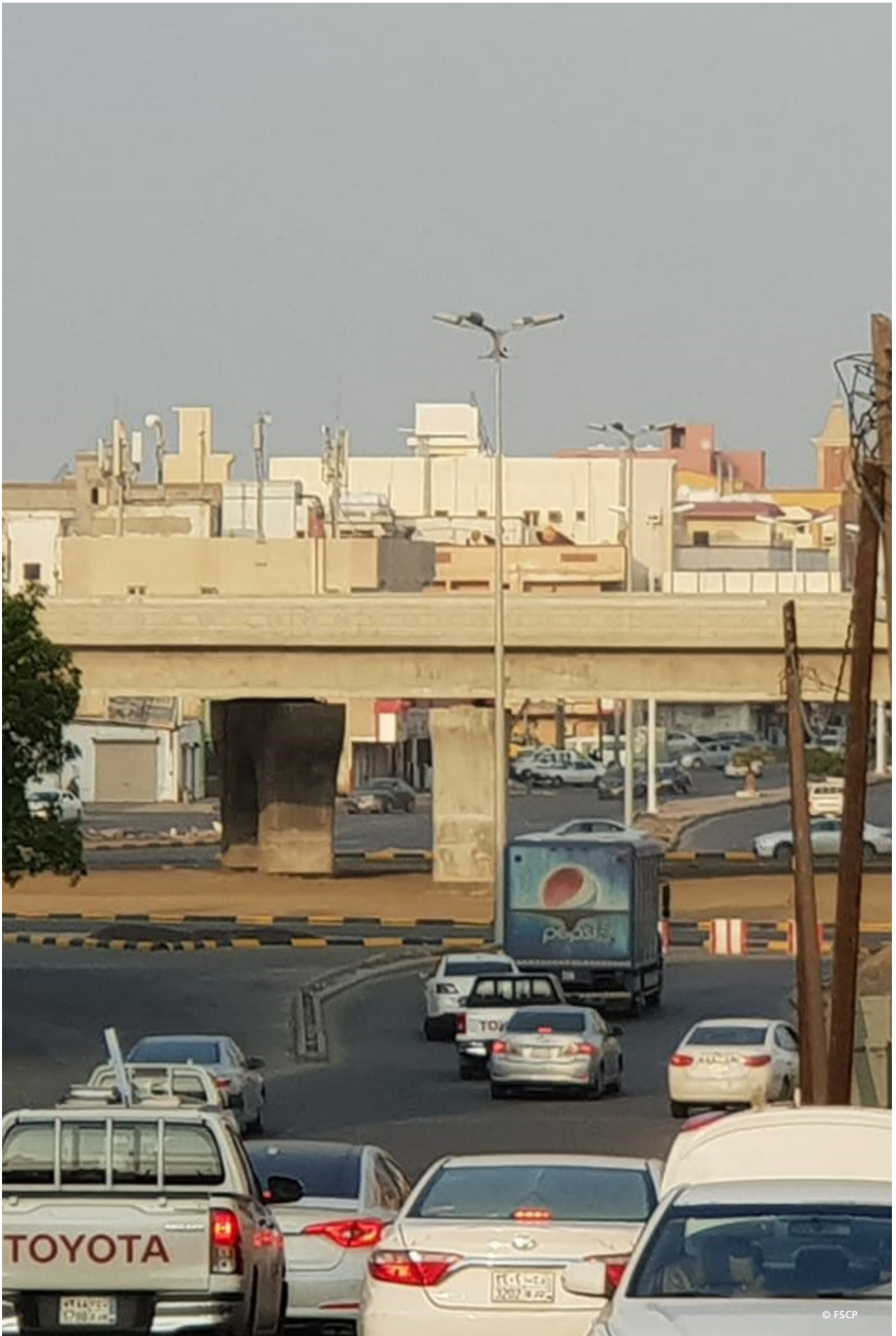
Central area along King Abdulaziz road
