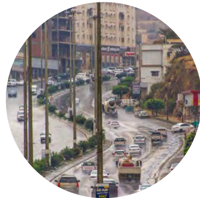
Overdimensioned infrastructure such as the regional roads divide the urban form and hinder coherent development
