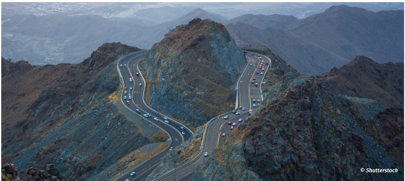
Al Hada Road from Makkah to Taif
