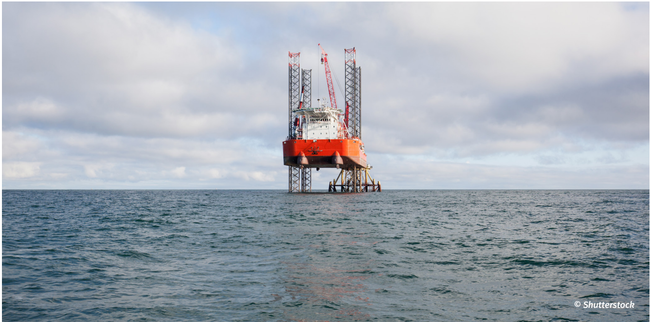
Oil platform in Saudi Arabia
