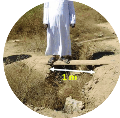
1. Earth fissures associated with water extraction
