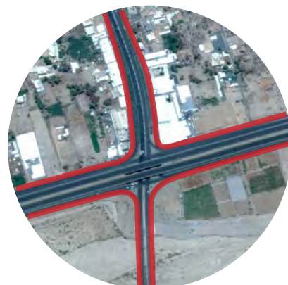
3. Overdimensioned road infrastructure
