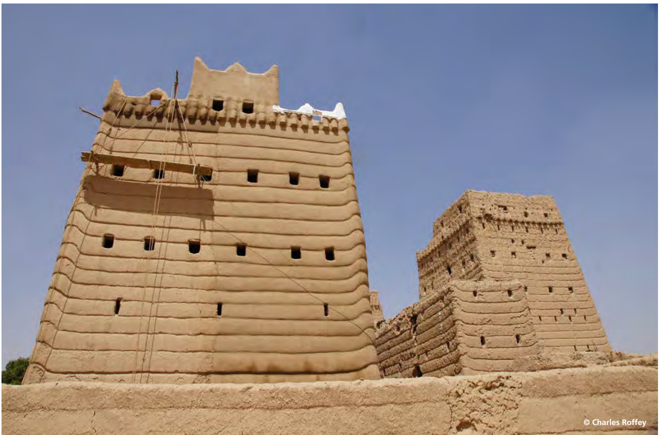
300 year old house in Najran under renovation
