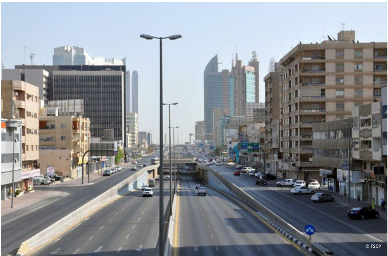
Roads infrastructure at the city centre
