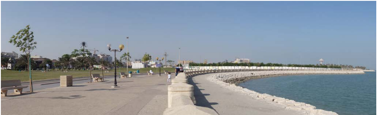
Current situation of the waterfront next to the port (Location C)
