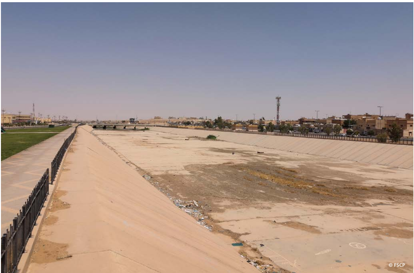
View from Wadi Arar inside the city
